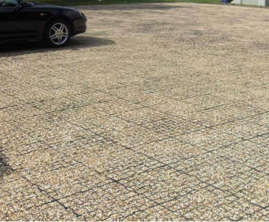
Geogrid is a high quality heavy duty ground reinforcement tile and cellular paving system.
